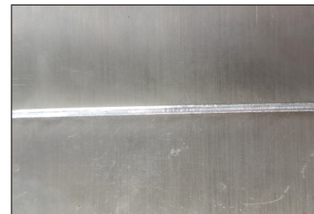
Stainless steel plate splicing
