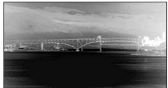
Showing highway bridge out 7.8 km using only TR4000 with 100mm lens
